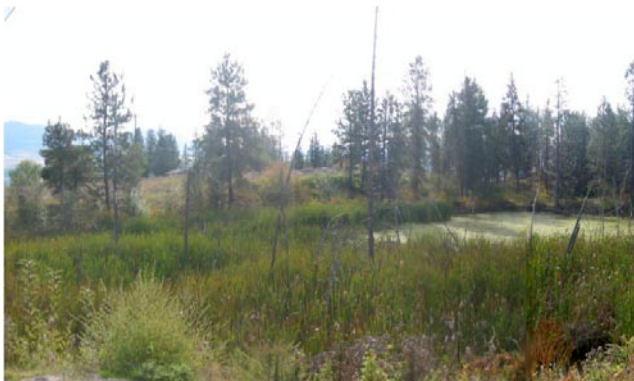
Existing Storm Detention Pond
