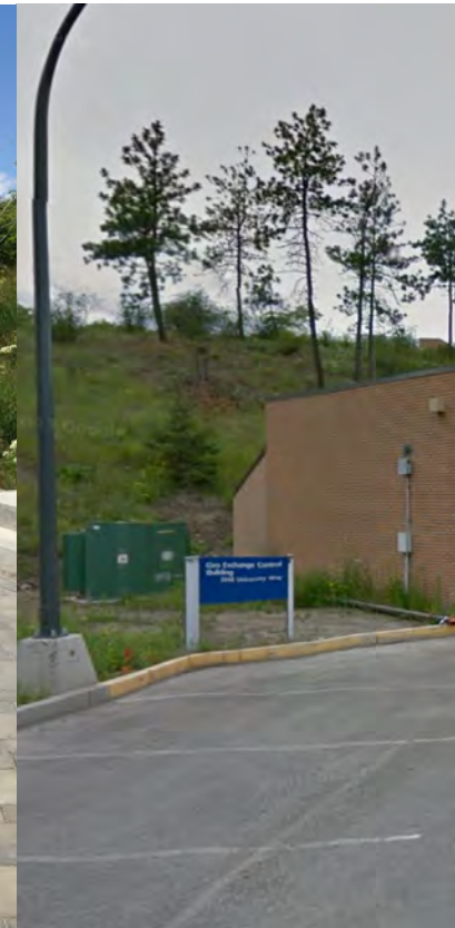
Geo Exchange Building
