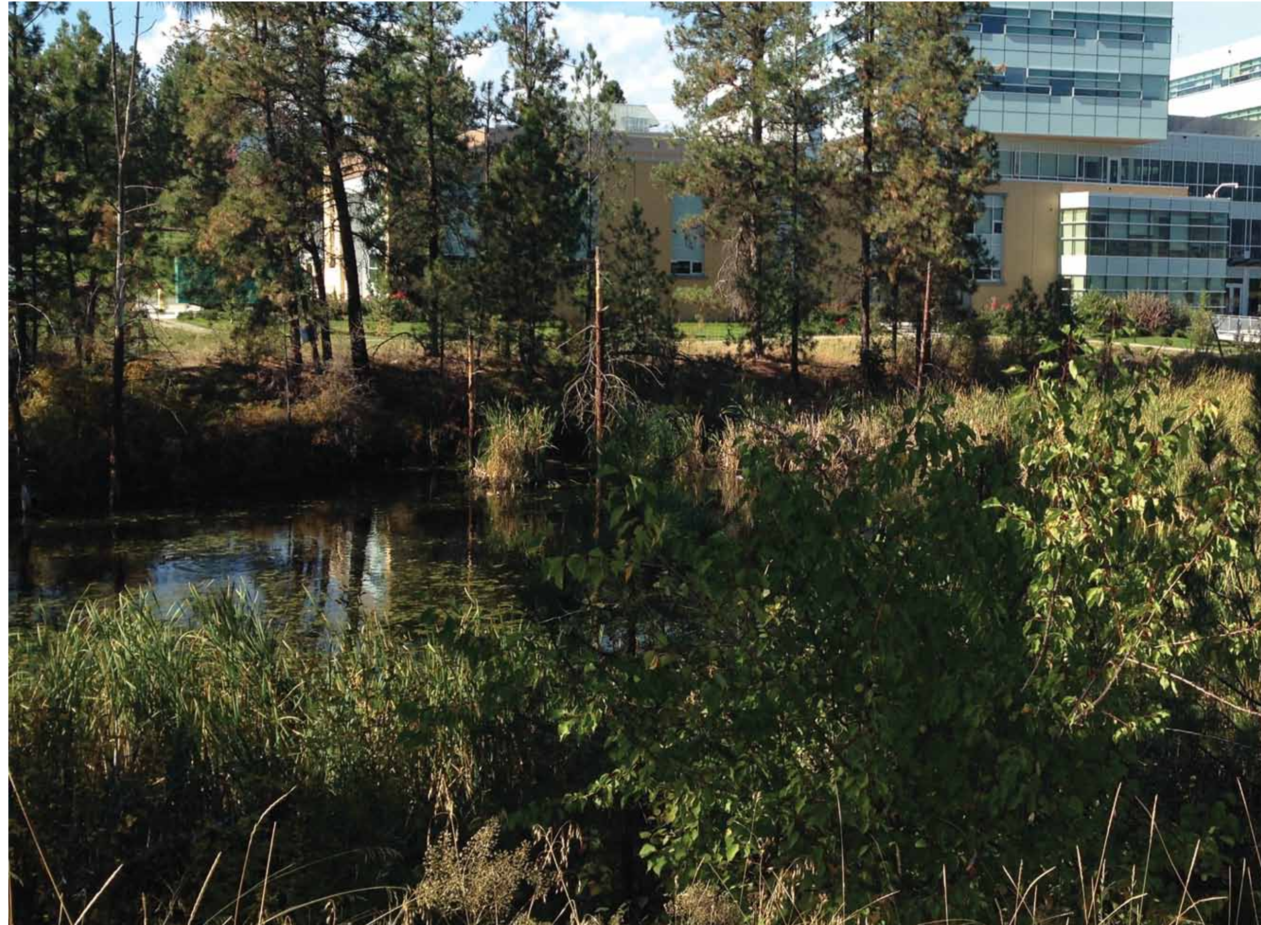
Stormwater Management Pond and Wetland
