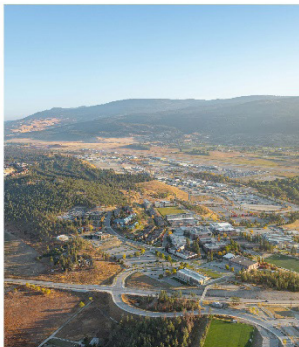
A new access to the campus from John Hindle Drive provides direct access for cyclists, pedestrians, and vehicles to the west side of campus.
